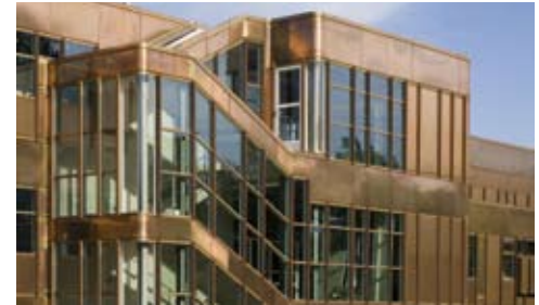
The building complex for the Humanities and Social Sciences has been completely reconstructed and now reflects a new image. Its reconstruction was part of a restoration process involving the entire central campus.
